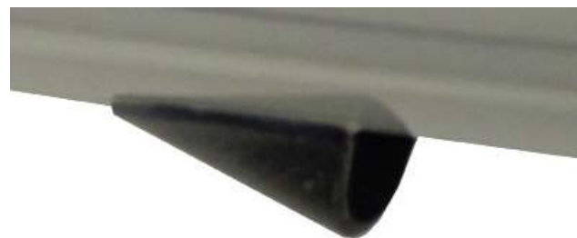
Carbon fiber scupper Installed
